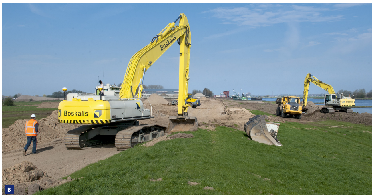
B Excavation work at the Tollewaard site
