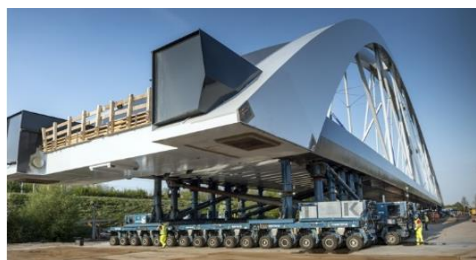
Figure 9 – Bridge just before transportation
