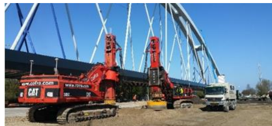
Figure 4 – Compaction operations next to the temporary bridge location
